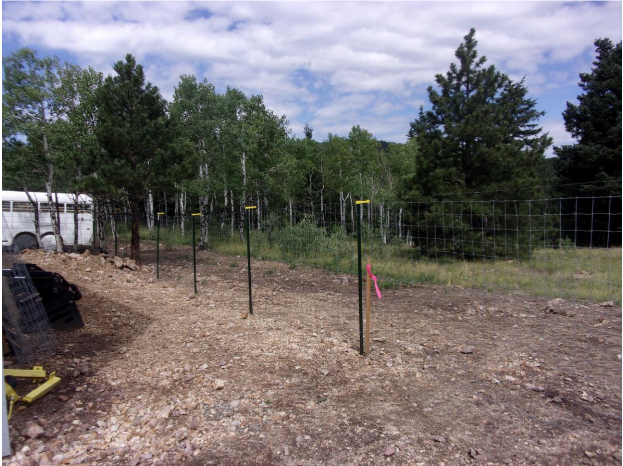
Fence at north property line, facing northwest
