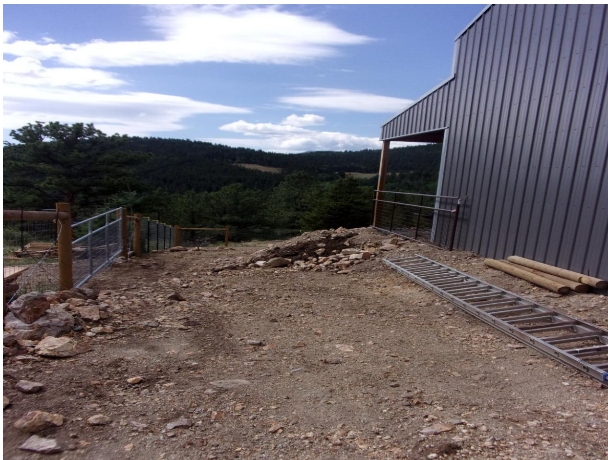
Eastern portion of barn, facing south
