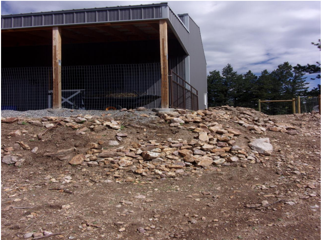
Eastern portion of barn, facing north
