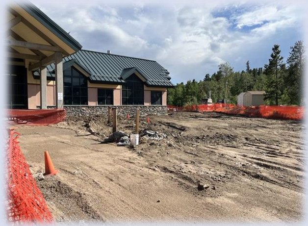
Regrading Project at Community Center
